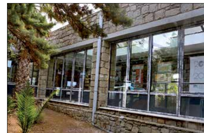
View of the building with the walls constructed of grey lava.
